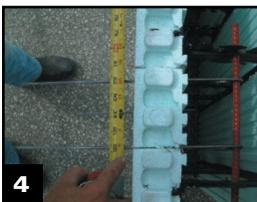
**6** Hook the connection ties on the web and slide into slits (fig. 4 & 5).
