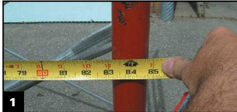
**1** Before starting the first course of forms the installer needs to measure the width of the frame scaffold being used for the tall wall adapter kit (fig.1).
