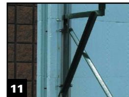
**12** Attach frame scaffold re-using connection ties, compression plate and self threading nuts.
