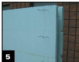
**7** Repeat steps 5 & 6 for entire first course and every course until the first pour height has been completed. Note: NUDURA Inc. recommends the height of the first pour not exceed the height of the box channel or frame scaffold dimensions.
